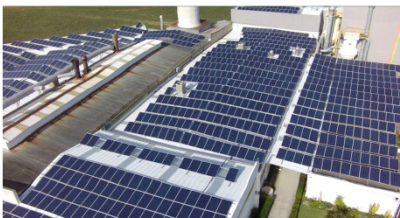
Fig. 1 Image of the roof installation on a factory-varying installation angles, roof outlets, different orientation to the sun, soiling (visible on the module rows in the background of the picture), changes of shading situations due to various roof installations
