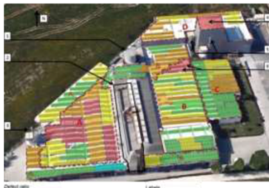
Fig. 1: Aerial picture of the roof installation of the investigated PV-plant on an industrial building. Positions of outlets emitting heat or dust are marked by the numbers 1 to 6. A, B, C, and D define different types of roof areas. The color code indicates the defect ratio of the strings [2]. (Imagery © 2017 Google, Map data © 2017 Google)
